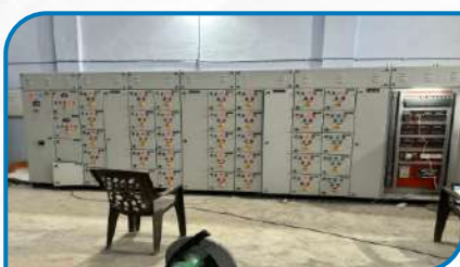
ELECTRICAL PANEL RETROFIT
